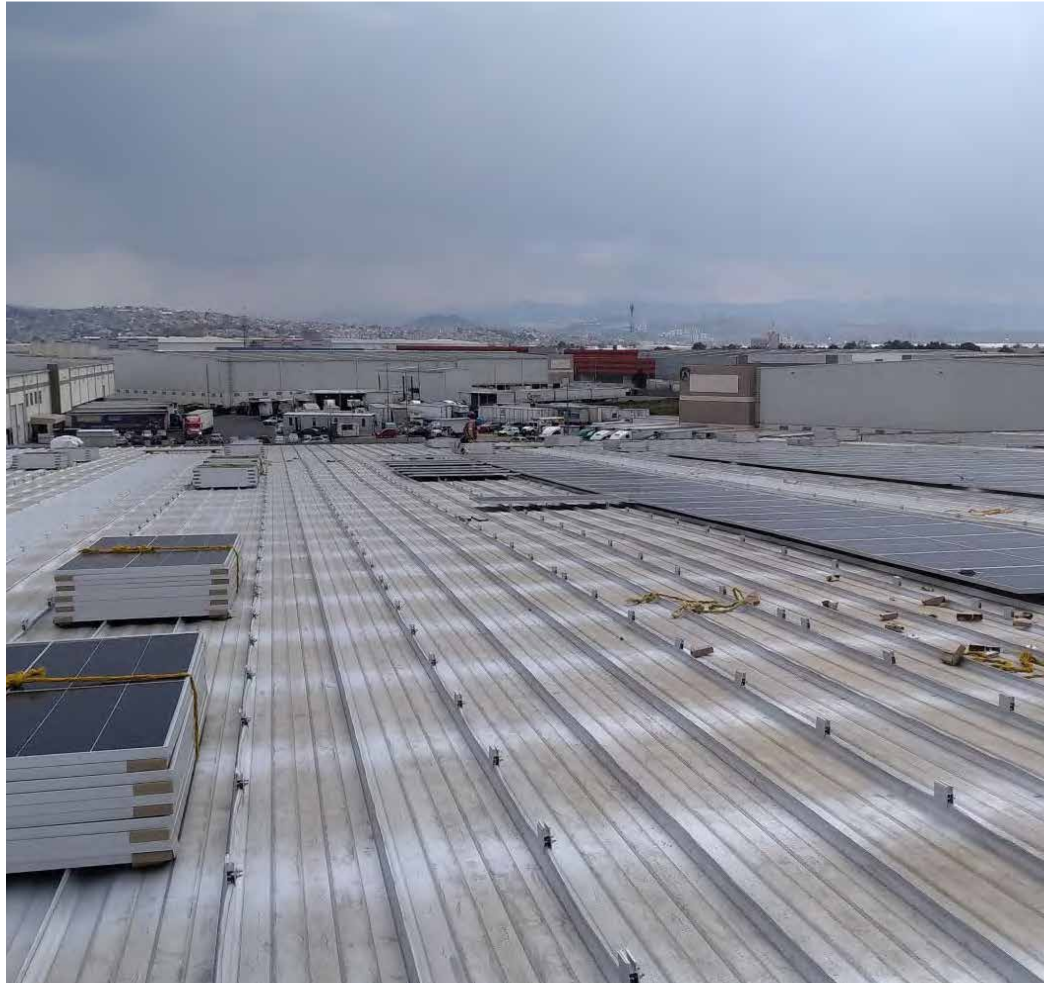
Solar panels being installed NIKE Mexico DC
