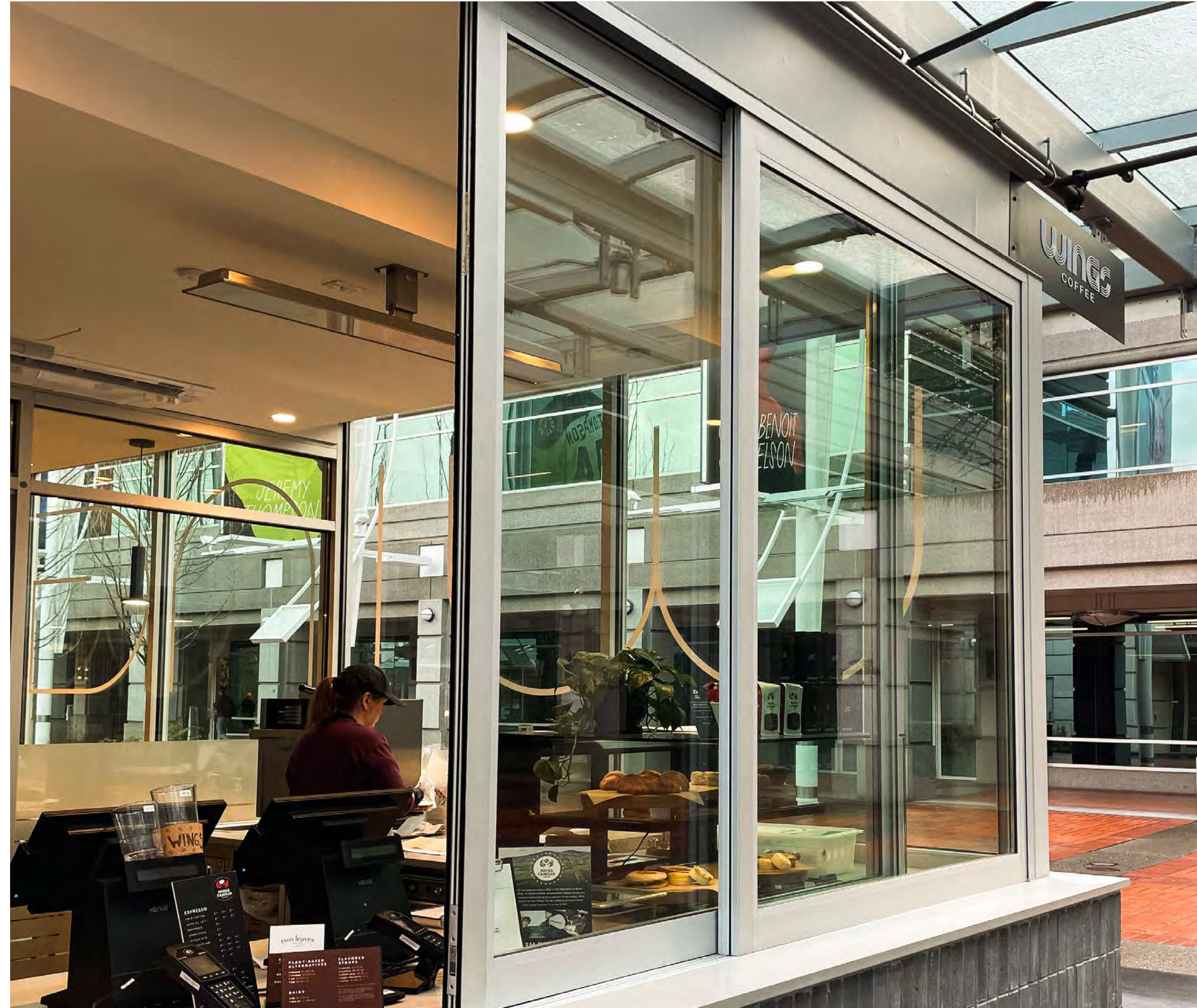
Wings Coffee located in the newly renovated Joan Benoit Samuelson Building at WHQ
